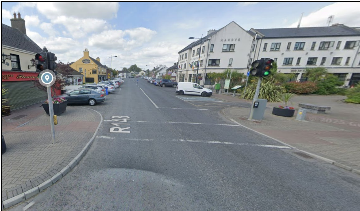
Figure 3.4: Pelican crossing with dropped kerb and tactile paving leading across Main Street (Source: Google Street View)
