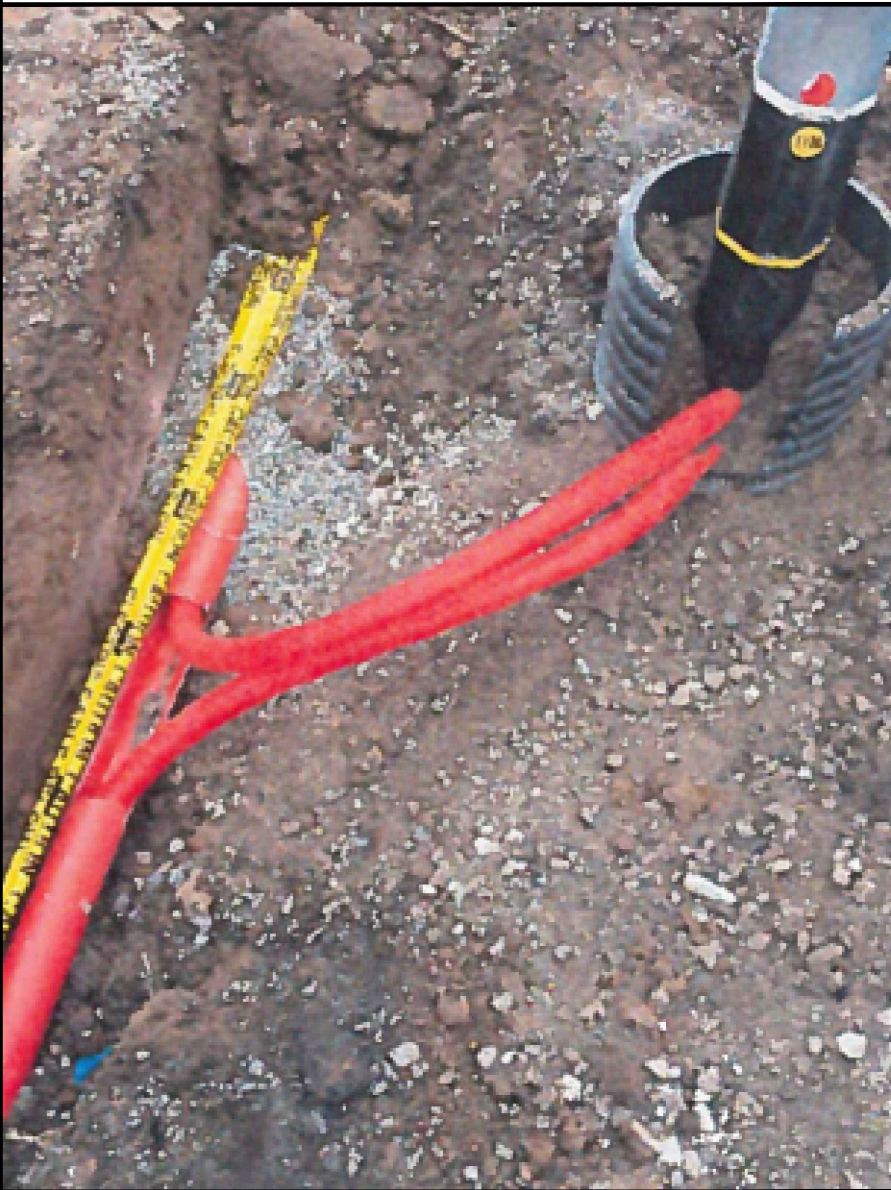
TYPICAL ARRANGEMENT FOR LOCAL DUCTING
