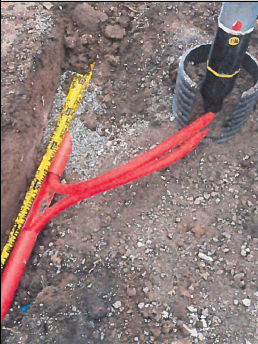
TYPICAL ARRANGEMENT FOR LOCAL DUCTING
